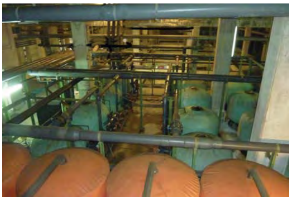
Conventional Sand Filters BEFORE (18 filters)
