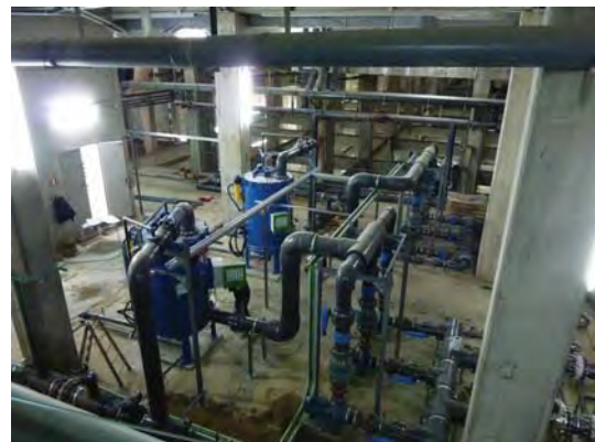
DEFENDER® Installation AFTER (2 filters)
